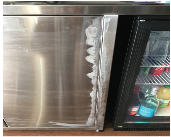
Extreme example of staining due to the weld cleaning solution residue not being completely removed/neutralised
